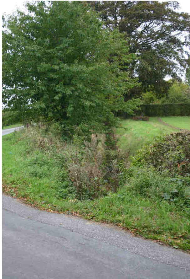
Fig 3 “Keldspring Beck” running alongside Keldspring Lane towards Barmby Moor [12]
