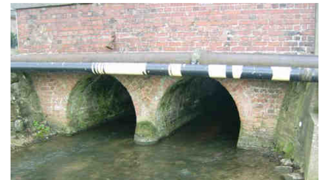
Fig 19 Double exit culverts along West Green Road
