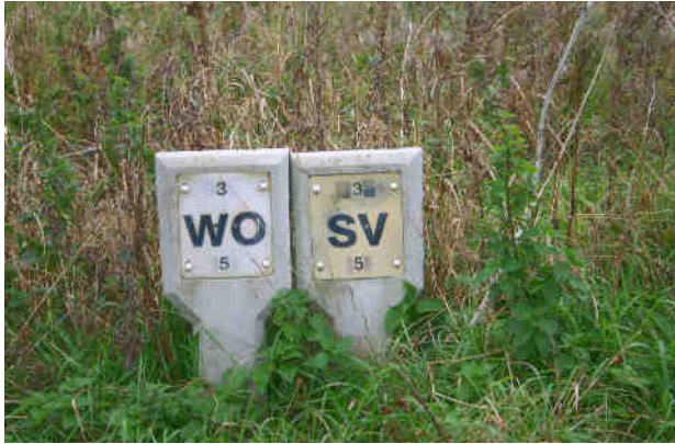
Fig 2 Water hydrants at Keldspring Lane [11]
